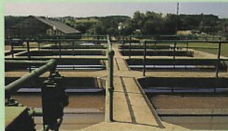
Sewage treatment plant
